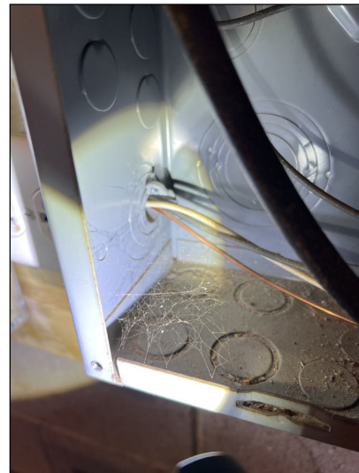
Broken/missing strain relief inside panel.
