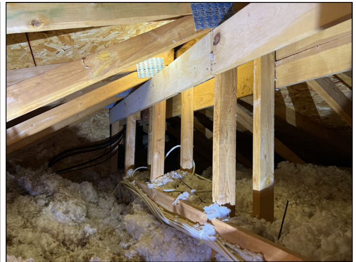
Appeared functional with no deficiencies noted at the time of the inspection.
