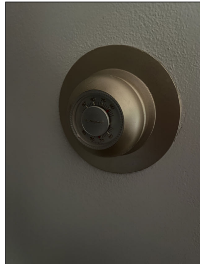
Functional at the time of inspection.
