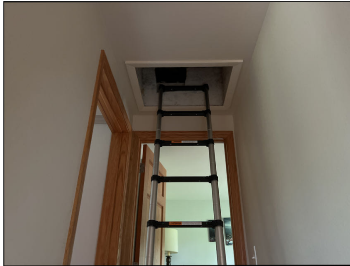
Appeared functional - with insulation over hatch door.
