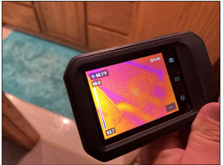
Radiant in-floor heating visible via thermal imaging
