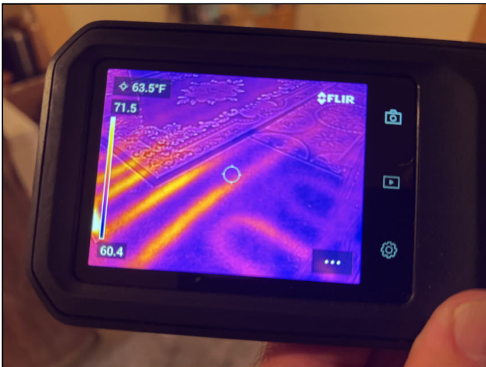
Radiant in-floor heating visible via thermal imaging
