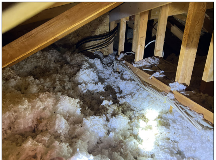
Insulation appears adequate.
