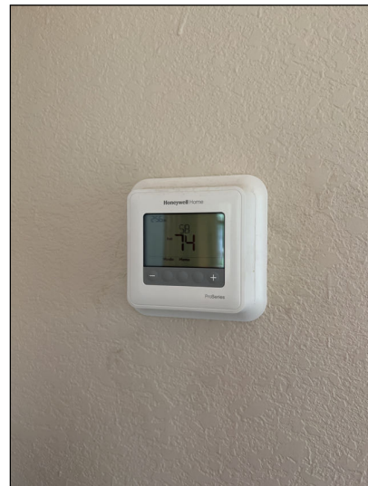
Functional at the time of inspection.
