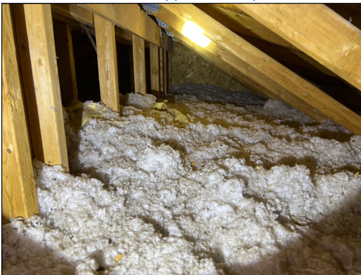
Insulation appears adequate.
