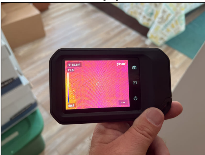
Radiant in-floor heating visible via thermal imaging
