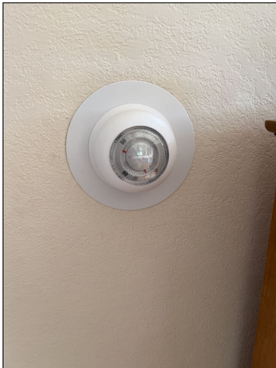
Functional at the time of inspection.
