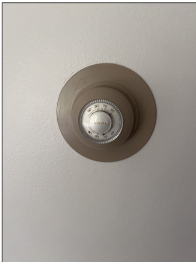
Functional at the time of inspection.
