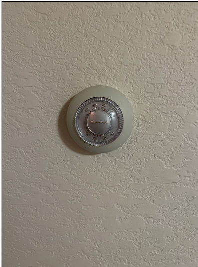
Functional at the time of inspection.
