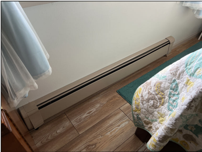
Radiators not getting warm in dining room, kitchen, and both main floor bedrooms. Possibly a bad zone switch valve. Recommend repair by qualified heating contractor.
