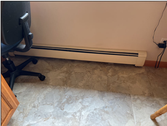
Radiators not getting warm in dining room, kitchen, and both main floor bedrooms. Possibly a bad zone switch valve. Recommend repair by qualified heating contractor.
